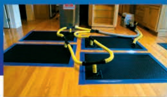
Hardwood Floor Drying
